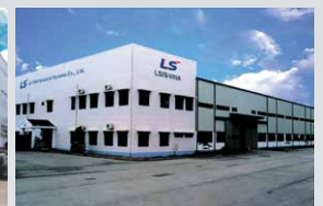
Hanoi factory (Vietnam) MV/LV switchgear, Mold TR
